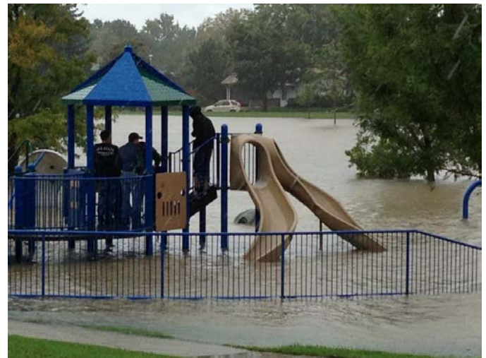
Utah Park in Aurora, Colorado is a detention basin that worked as designed to minimize damage from floodwater to neighboring property during the September, 2013 flooding.
