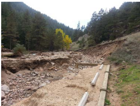
New channel cut by Fourmile Canyon Creek in Boulder County near UDFCD border. Actual creek channel is left of photo. Damaged parking area served the Anne U. White Trailhead prior to the flood.
