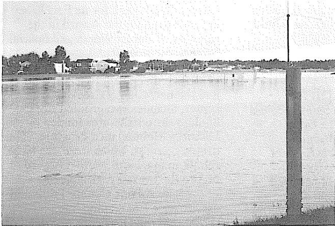
Expo Park on Westerly Creek in Aurora on June 6, 1991. Detention in a park. Note the ball field back stops in the center of the picture and the ALERT gage standpipe in the right foreground.
