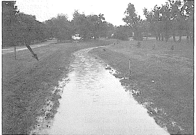
High water line on a grass lined channel on Westerly Creek in Montview Park in Aurora from the June 6, 1991, event.
