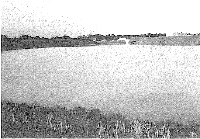
Kelly Road Dam, normally dry, on Westerly Creek on June 6, 1991.
