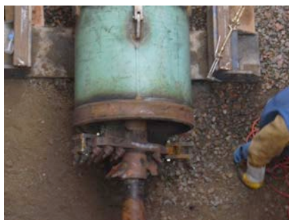
Thirty-inch casing and auger
