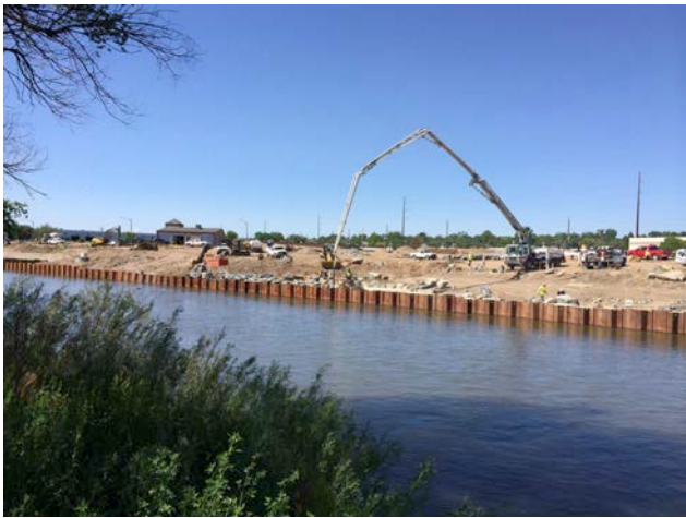
Johnson – Habitat Park under construction
