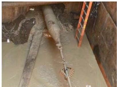
Fourteen-inch fusible PVC and ream
