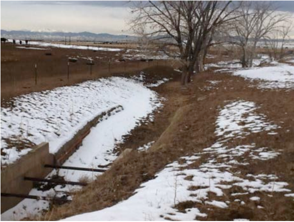
Pre- and post-construction of Bolling Drive Tributary
