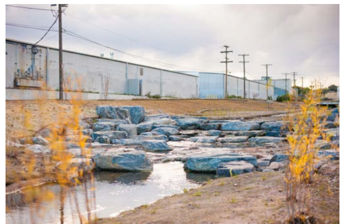
Drop Structure on Weir Gulch
