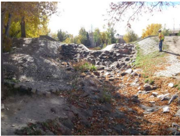
Pre- and post-construction spillway
