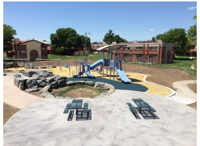
Completed Playground at Weir Gulch
