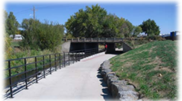
Coal Creek at 120 th after construction.
