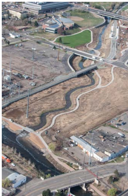
Completed Lower Lakewood Gulch Reach
