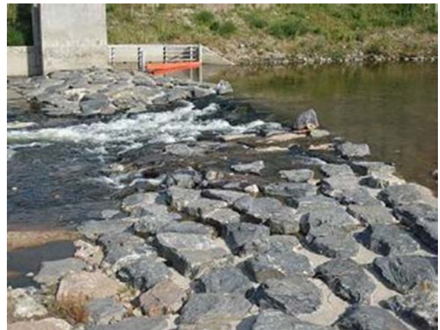
New Diversion Dam with boat chute
