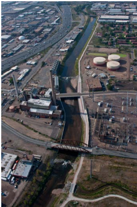
Completed South Platte River Reach
