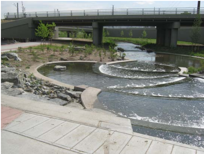
Completed Lakewood Gulch Ring Drop
