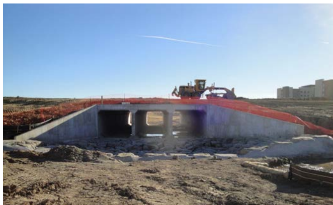
Drainage structures for the East Corridor CRT to DIA went in very quickly in late 2012.
