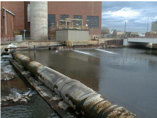
Old Inflatable Diversion Dam at Zuni Power Plant
