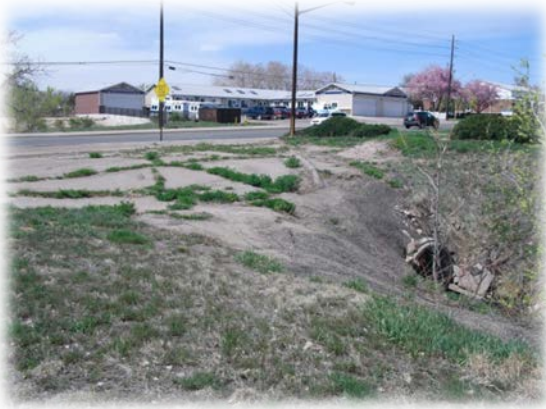
Existing Grange Hall Creek crossing
