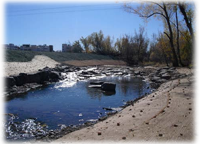
Boulder Creek drop structure and fish passage.
