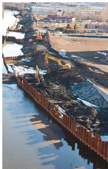
Sheet pile water control within the South Platte River
