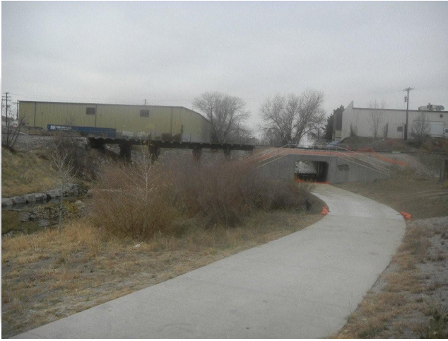
Views of the West Harvard Gulch project.
