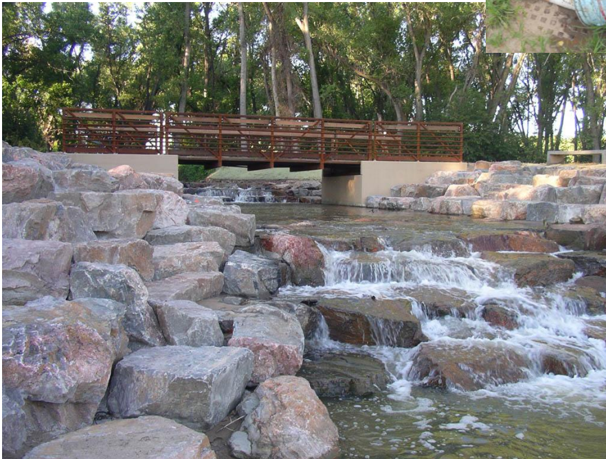
Finished drop structure looking upstream at Marcy Gulch. (Inset) Trout caught in Marcy Gulch
