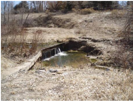
Check structures (left) had been installed to keep potential degradation to a manageable level (center and right)
