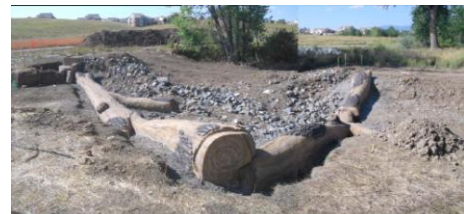
Concrete log drop during construction
