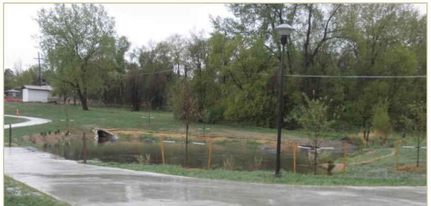
Richey Park detention after construction, looking downstream at the pond outlet and upstream at the forebay
