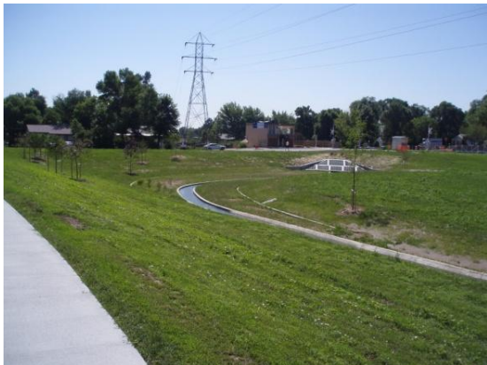
Richey Park detention after construction, looking downstream at the pond outlet and upstream at the forebay
