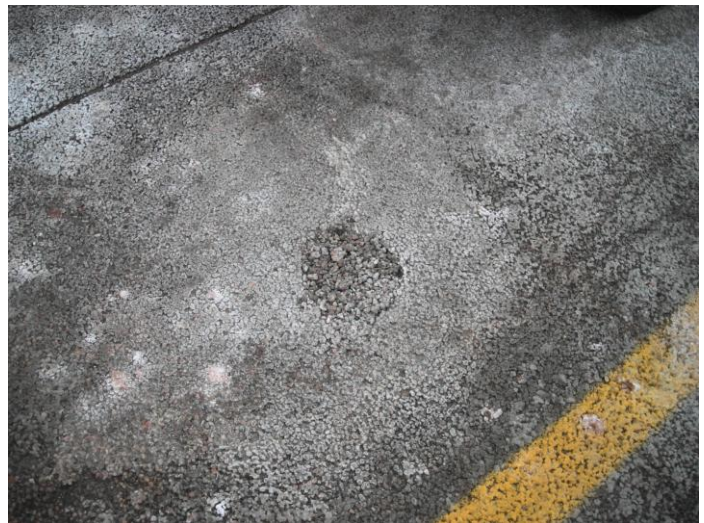
Photograph 2. In December 2009, the section with small aggregate started to ravel. It spread quickly, by January 2010 a number of areas showed raveling in excess of 2 feet in diameter.
