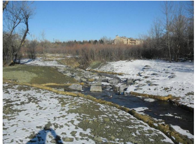
Looking north at improved corridor, partially grouted drop structure stabilizes the channel and protects upstream wetlands
