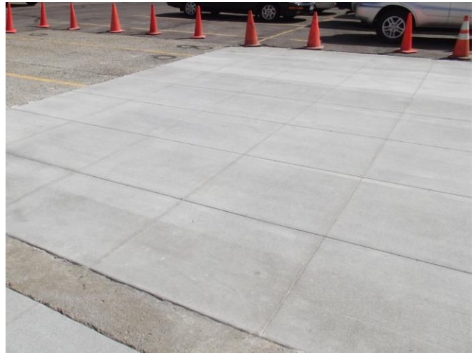
New permeable pavement test pad in Lakewood
