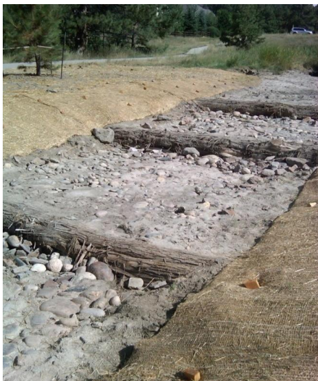
Timber drop structures immediately after construction.
