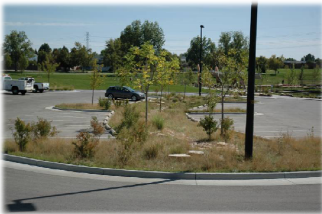
Bio-swale treats parking lot runoff before entering lake.
