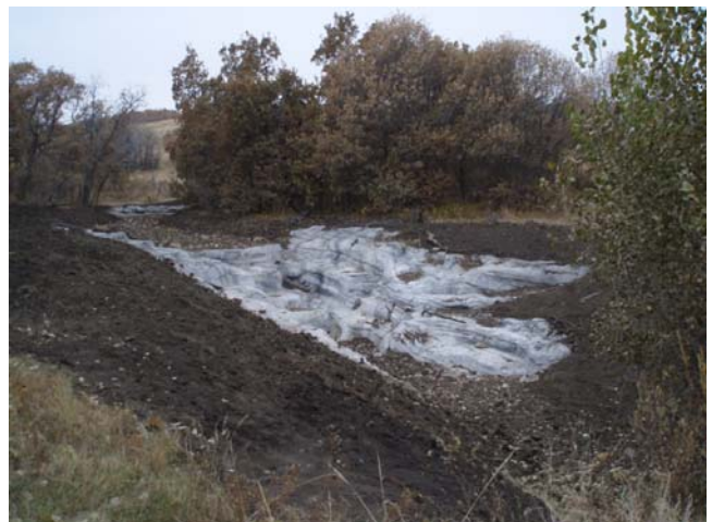
After – Oak Hills Tributary in Castle Pines North
