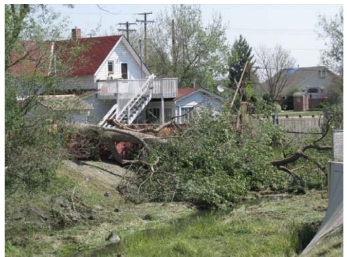
Lena Gulch – Example of the hail and wind storm damage in Wheat Ridge.
