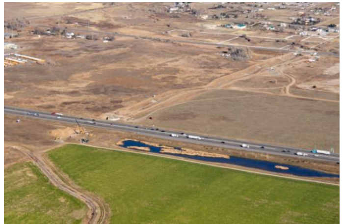
McKay Lake Drainageway, phase one channel construction nearing completion between I-25 in the foreground and Washington Street in the background.
