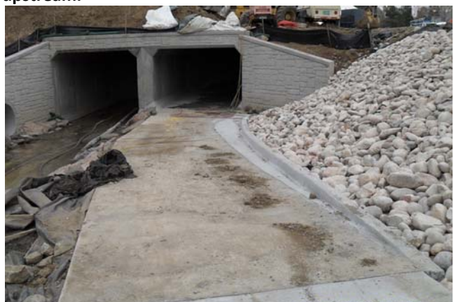
Near Completion – Same view at Arapahoe Road.
