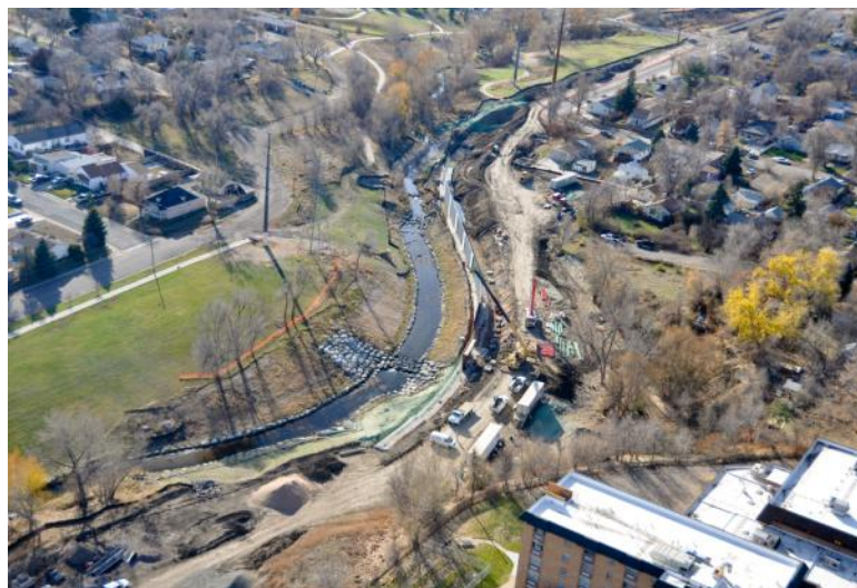
Drop Structure No. 2 on Lakewood Gulch west of Knox Court in the "Oxbow Area"
