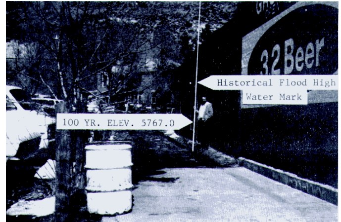
Bear Creek flood levels in Morrison between Market Street and Mount Vernon Street downstream of the Mount Vernon Creek confluence. The “Historical Flood High Water Mark” depicts the level of the September 2, 1938 flood.
