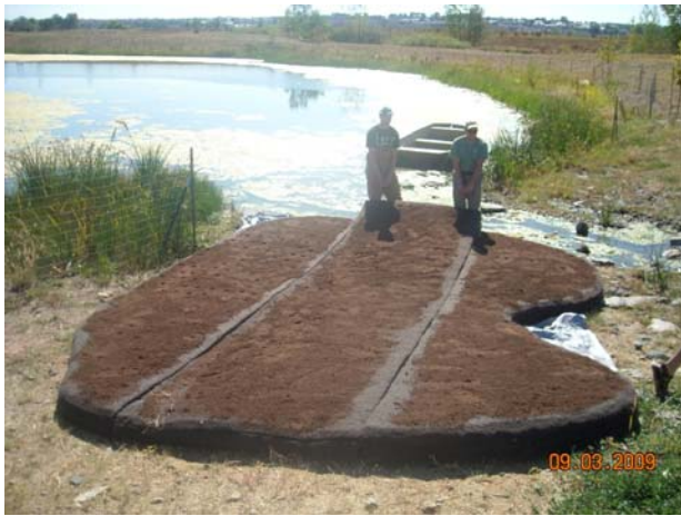
Floating Island during installation
