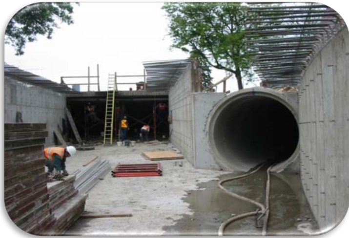
Construction of diversion structure to existing brick storm sewer
