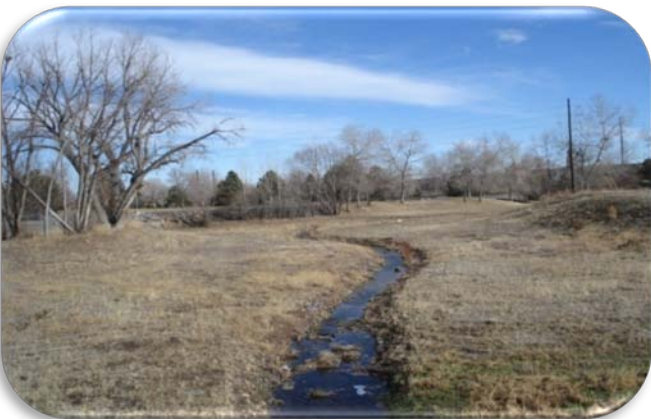
Lena Gulch at Isabell, looking downstream from the boulder drop structure which is downstream of the box culvert under Isabell Street
