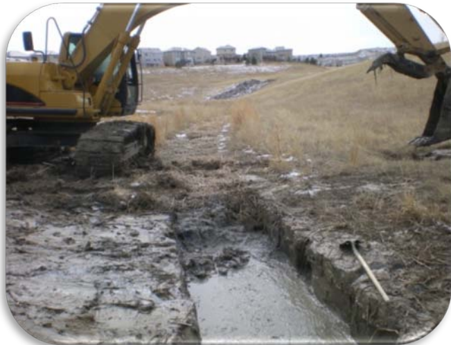
Community Drainageway West during sediment Removal operations
