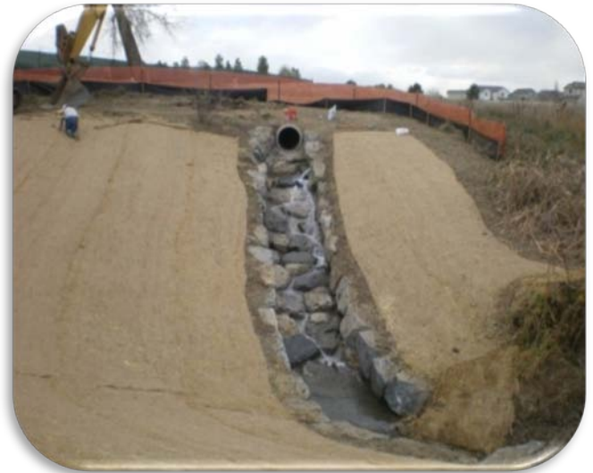
Windmill Tributary, grouted boulder rundown, after construction
