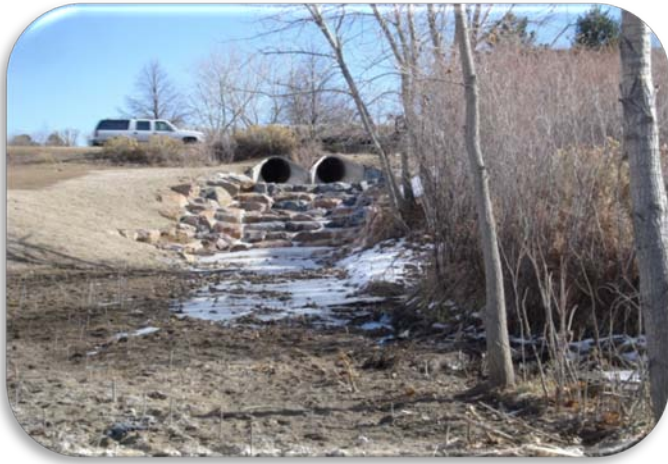
Dad Clark Gulch, Unnamed Tributary, looking upstream toward the twin 48-inch CMPs
