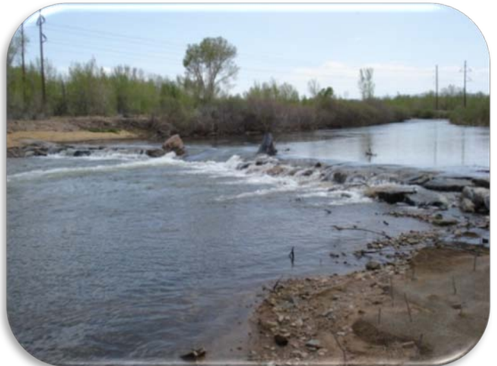
South Platte River after repairs
