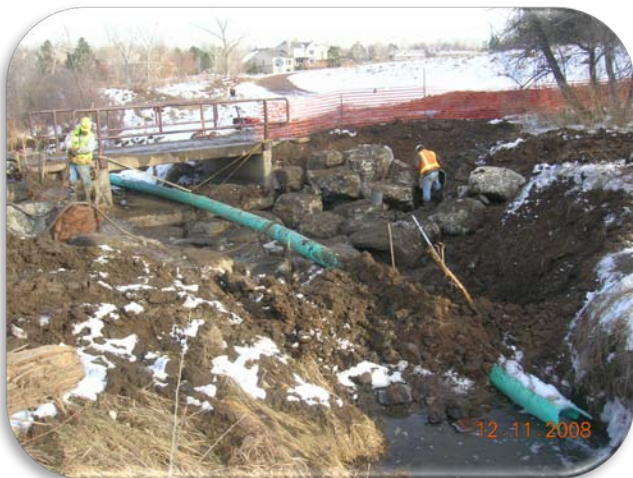
Water control is a major project element on Lee Gulch as a drop structure is rebuilt and the trail stabilized
