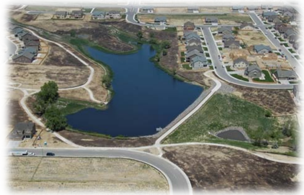
Marshall Lake Dam, flood control was provided above the permanent water surface as a result of dam rehabilitation under the supervision of State Engineer's Office. Horizon Tributary to Brantner Gulch was stabilized throughout this development. 136 th Avenue is visible in the background.
