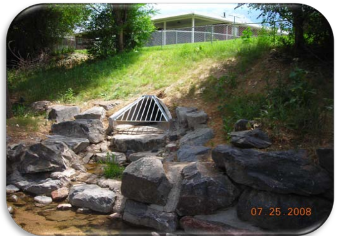
The 36-inch storm sewer outlet to Big Dry Creek is protected from erosion with grouted boulders
