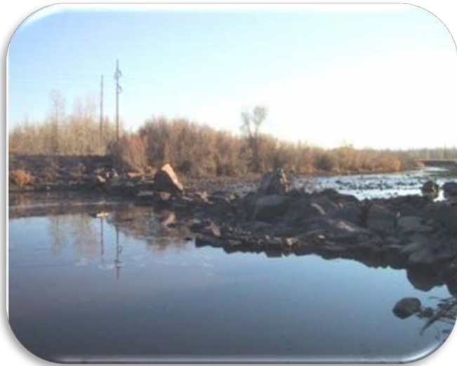
South Platte River rock weir before repair
