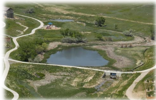
Villages at Riverdale regional water quality pond. An existing agricultural pond was rehabilitated with a new water quality outlet structure and discharge pipe, embankment repairs and high level outlet control. The trail crossing is above the 10-year water surface, more infrequent discharges overtop the trail. The forebay is visible upper-left. The area between the forebay and dam embankment was not disturbed.
