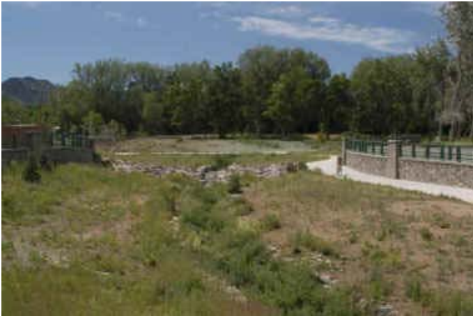
Looking upstream, showing the decorative walls, trail and grouted boulder drop structure
