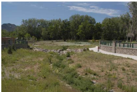
Goose Creek channel, decorative walls and trail
