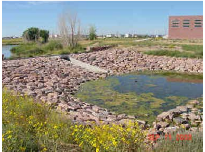
Parkfield Lake spillway in Denver
