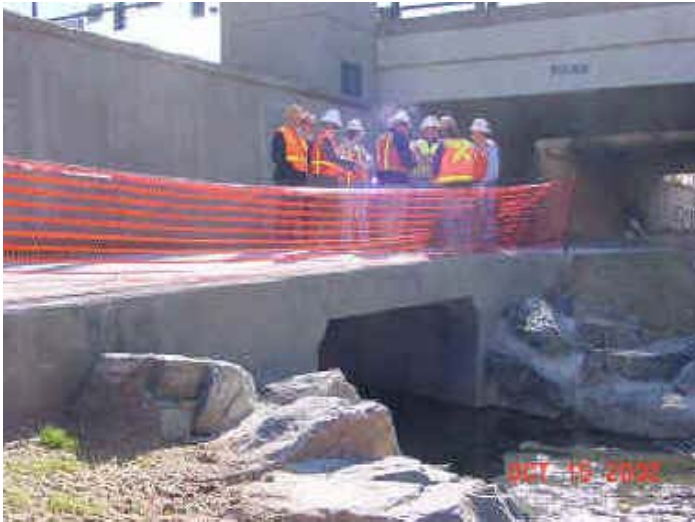
Convention Center storm sewer outlet to Cherry Creek in downtown Denver
