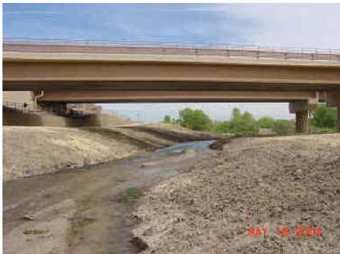
Bronco Parkway bridges over Cherry Creek in Arapahoe County
