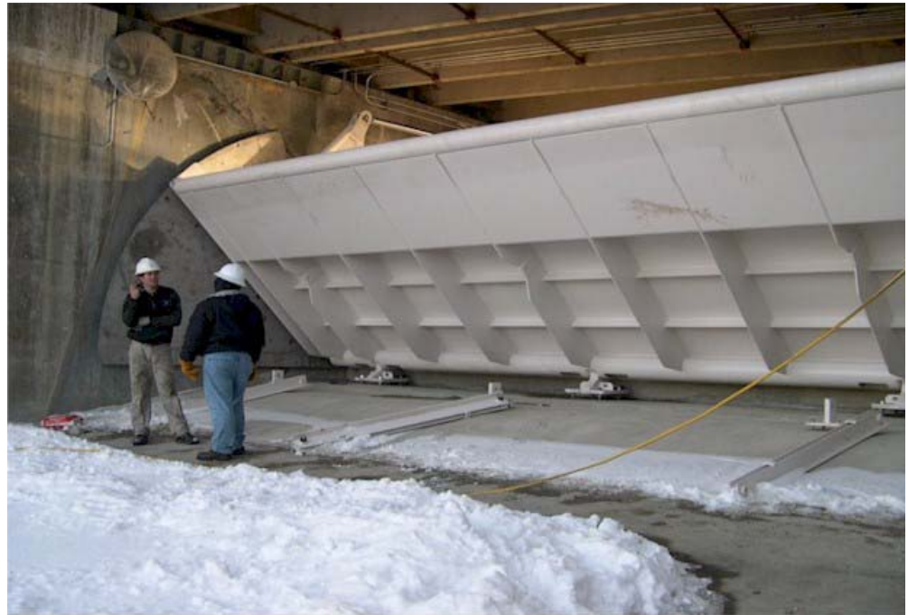
Looking upstream at one of the new gates
