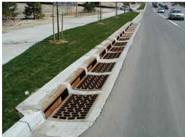
Inadequate or overkill? These Denver No. 16 combination inlets were sized using the HEC-22 method.
