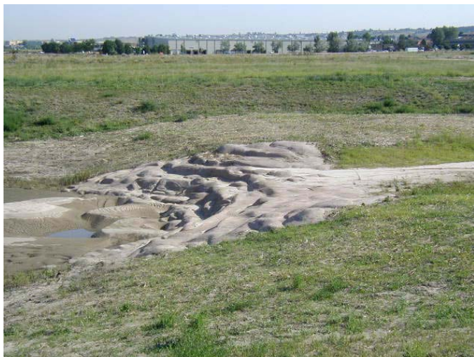
Long's Way Tributary sculpted concrete drop structure.
