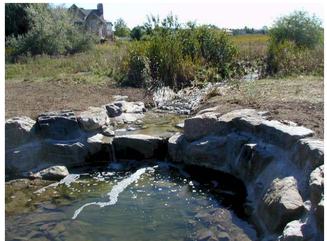
Greenwood Gulch drop structure. The sheet pile cutoff wall is hidden behind the grouted boulder drop structure.
