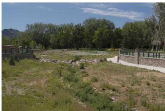
Goose Creek channel, decorative walls and trail
