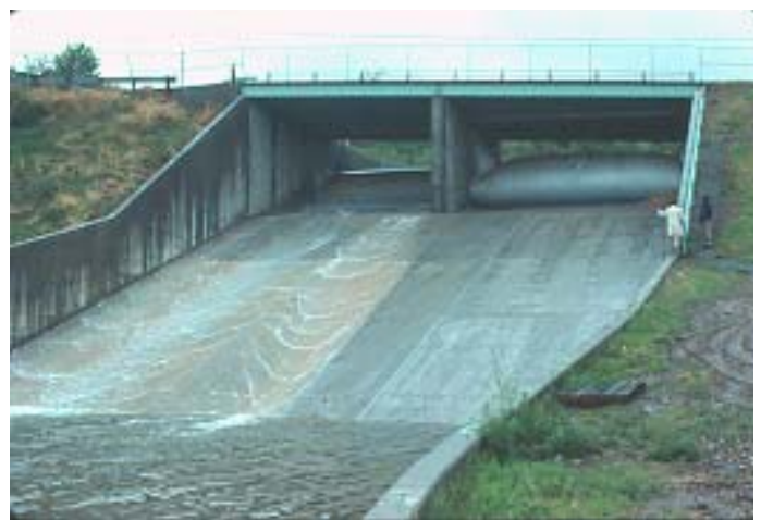
Looking upstream at the old fabridams
