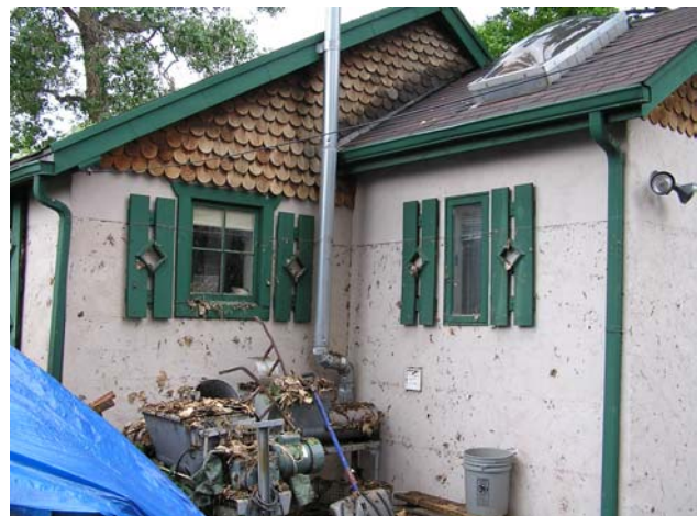
High water mark on home in Golden
