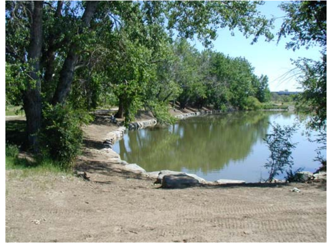
Overland Pond – After. Note vertical boulders protecting trees and trail.
