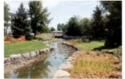
Immediately after construction
