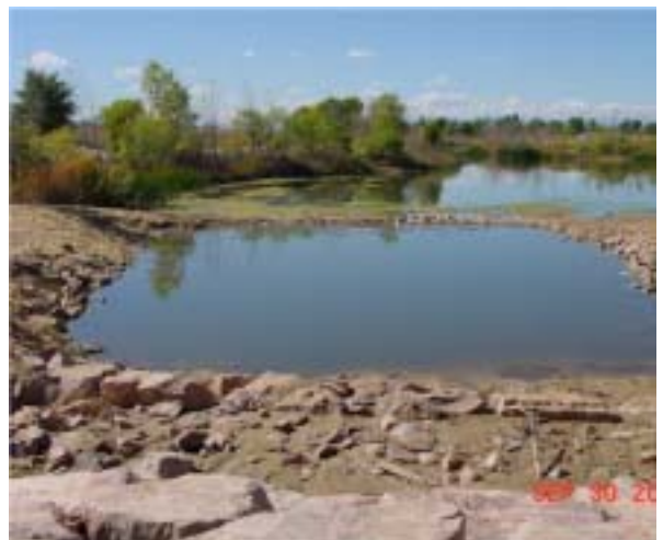
Parkfield Lake inlet channel forebay.
