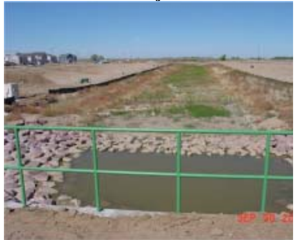
Parkfield Lake outlet channel.
