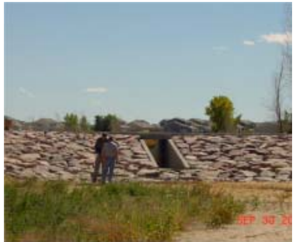
Parkfield Lake spillway.
