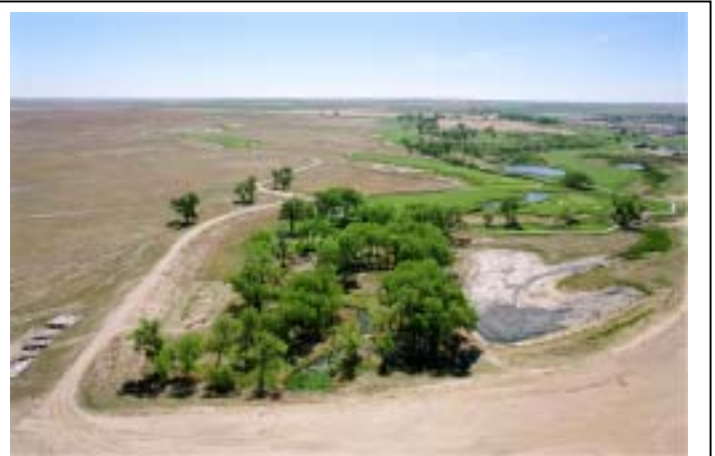
Last year I wrote about the completion of the Green Valley Ranch Golf Course detention facility. Here is an aerial view showing the road embankment that creates the detention, the creek, a water quality pond for local runoff and portions of the 16 th and 17 th holes.
