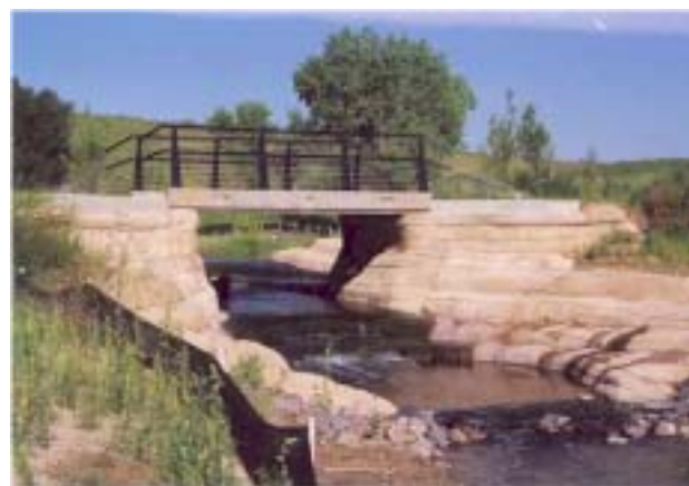
Two of the Grange Hall Creek sculpted structures.
