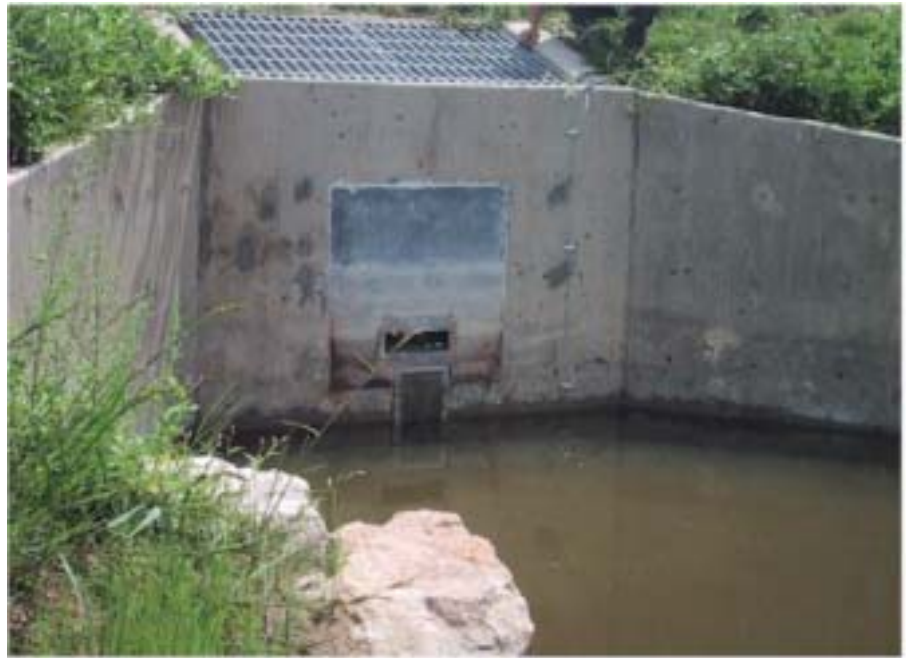
Figure 1. Extended detention outlet installed June 2001 in operation in August - 18 hours after storm's end. Note the partially submerged well-screen type trash rack, the debris line that is near the bottom of the 10-year control orifice and the 100-year overflow on top.
