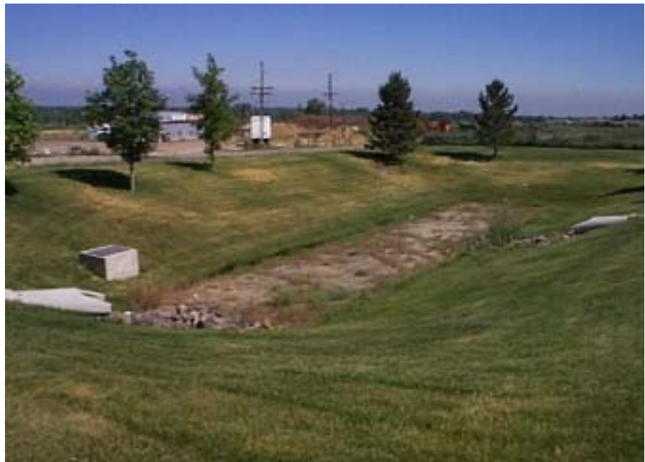
Figure 2. Sand filter with water quality capture volume above it, installed late 1980s. Note two inlet pipes and an overflow for larger storms. Volumes below the overflow are filtered and, because site conditions permit, infiltrated into the ground.
