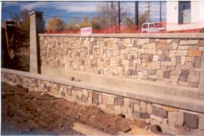
Goose Creek form liner detail.
