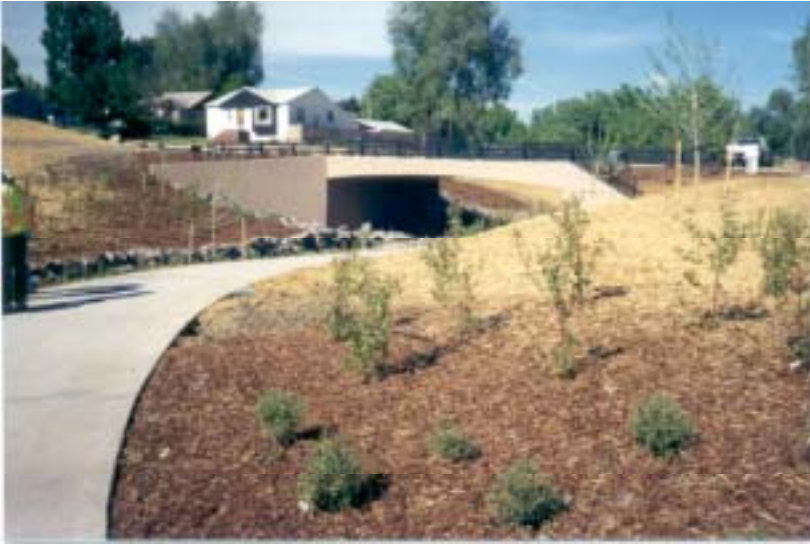
Looking upstream at the new Perry Street bridge along Lakewood Gulch.
