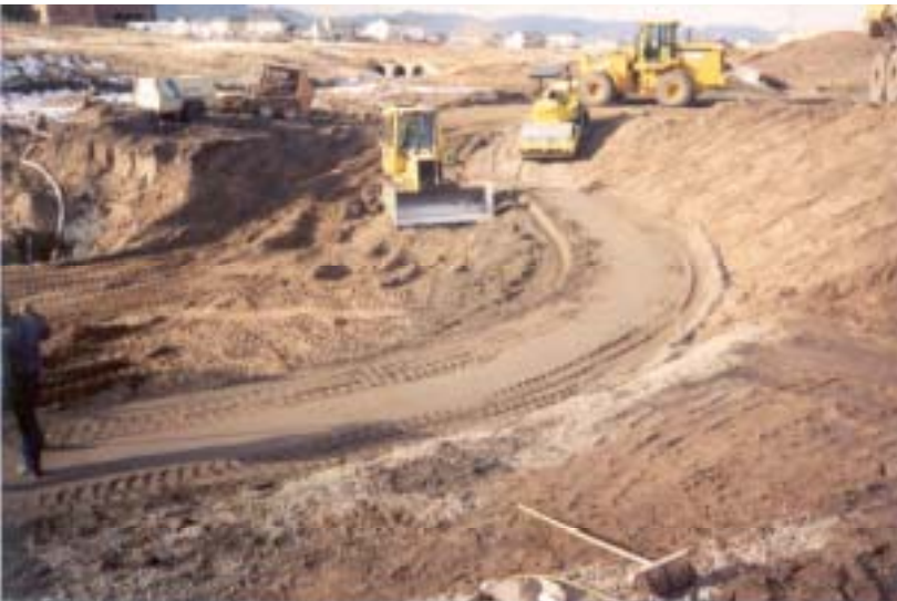
Constructing a soil cement drop structure on Marcy Gulch.
