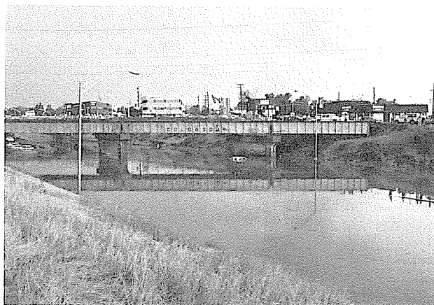
Figure 3. I-25 at Evans Ave. on July 20, 1992.
