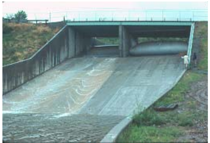
Looking upstream at the old fabridams
