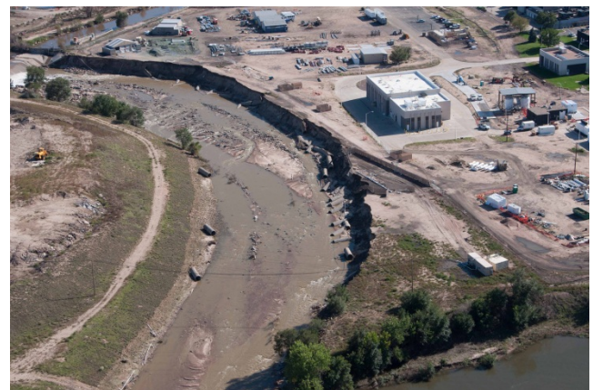
Flood waters on Sand Creek at the confluence with the South Platte River eroded approximately 100 feet of the outside bend into the Metro Wastewater Reclamation plant property, leaving a 25 foot vertical bank.
