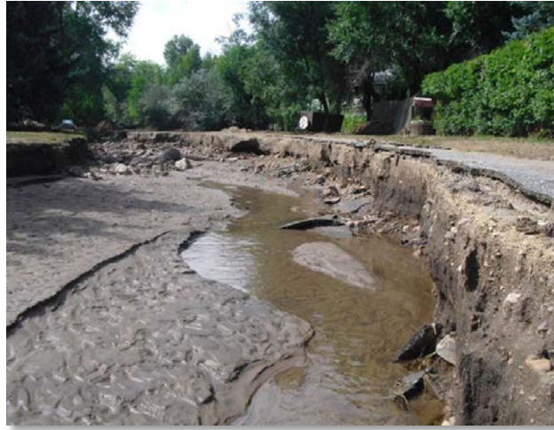
Fourmile Canyon Creek in Boulder, CO reclaimed its natural easement in what was previously a residential street and front yards during the September 2013 flooding. A major drainage system was planned for this creek but not implemented before the flood.
